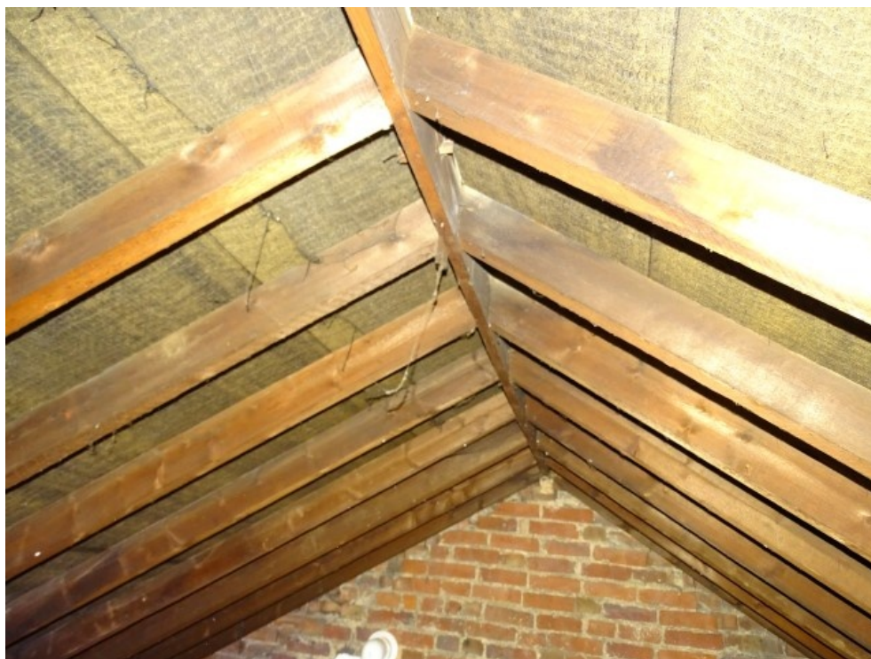
General view of roof structure
