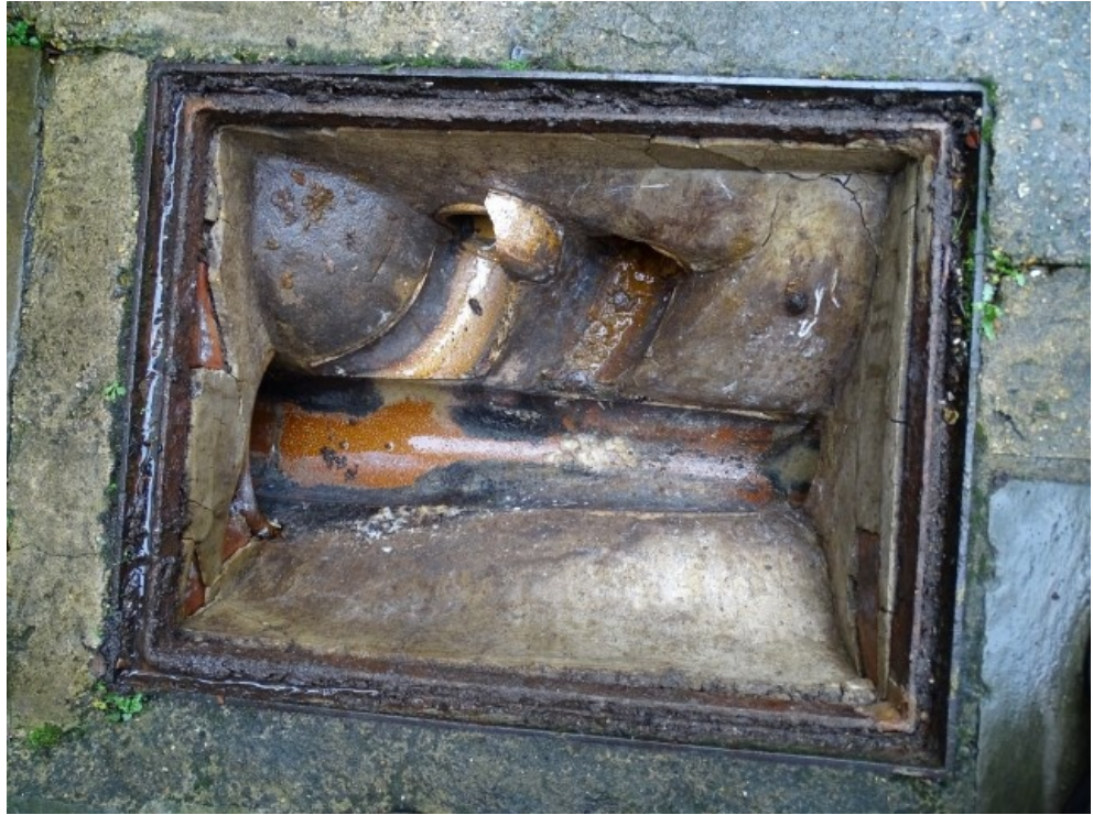
Main drain in alleyway
