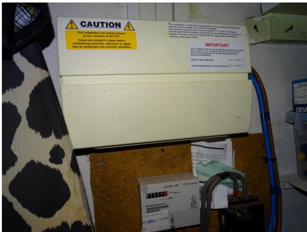
Electric meter and consumer unit
