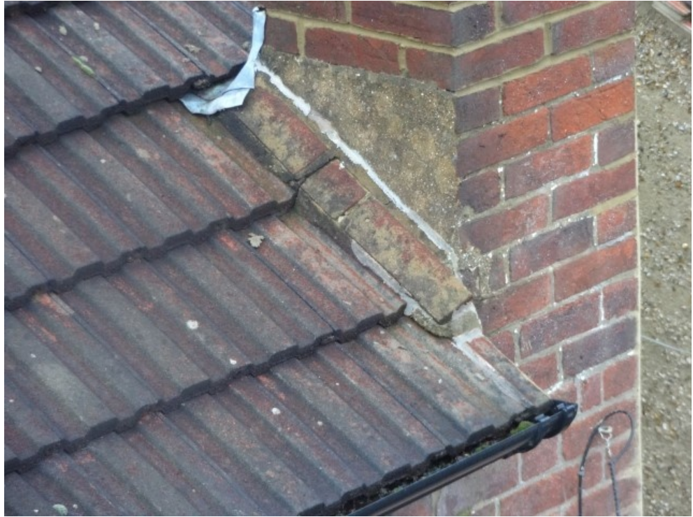
Tiled flashing to chimney stack
