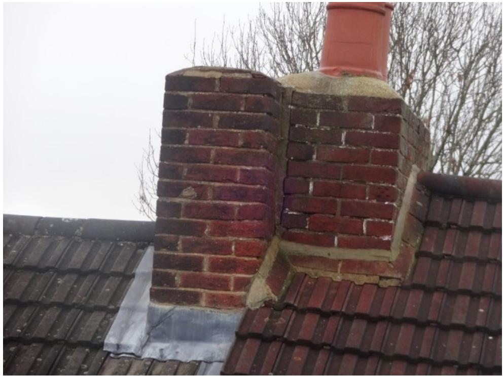
Main chimney stack
