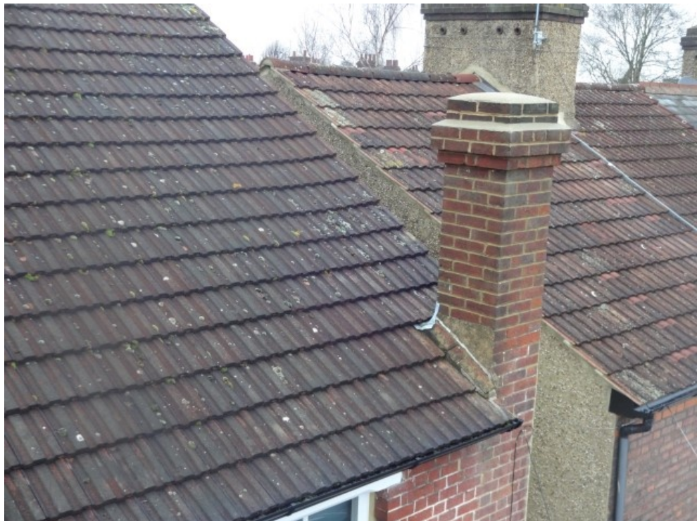
Front bedroom chimney stack
