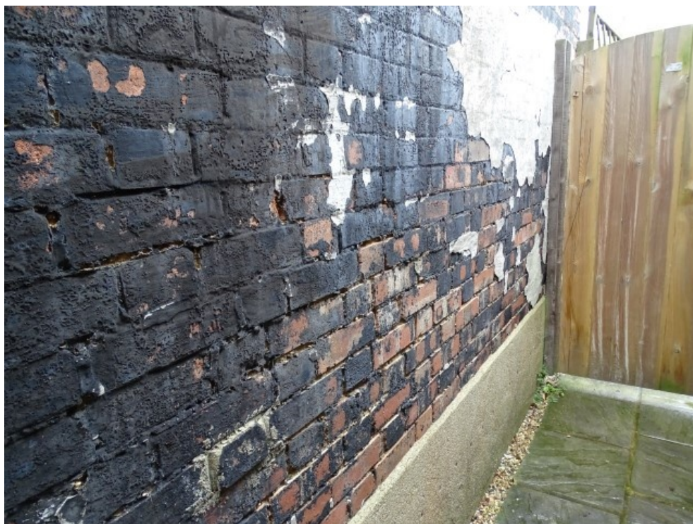
Rear gable wall right hand side rear of kitchen
