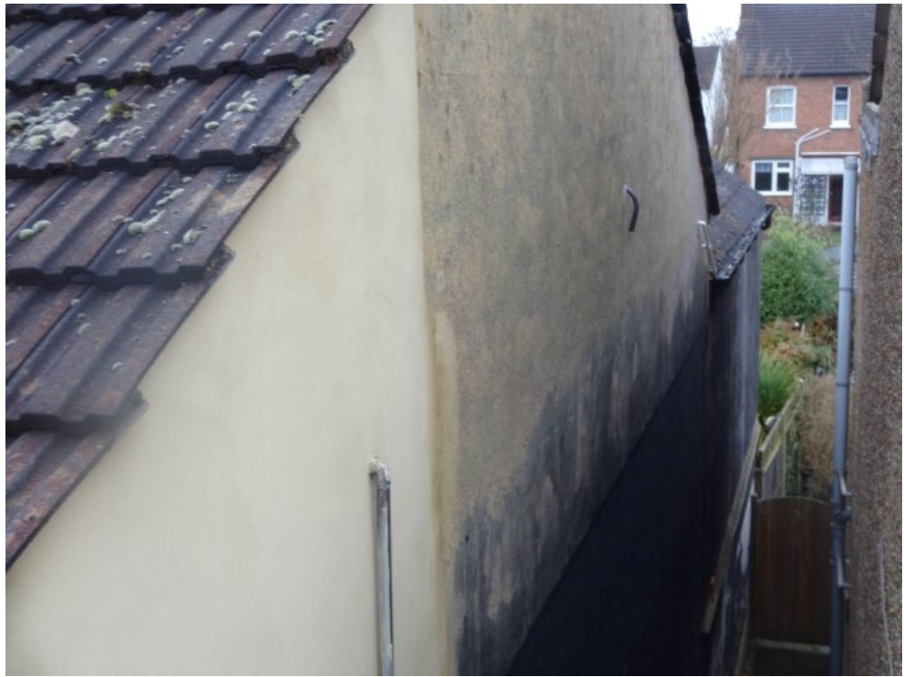
Right hand gable end rendered down to first floor
