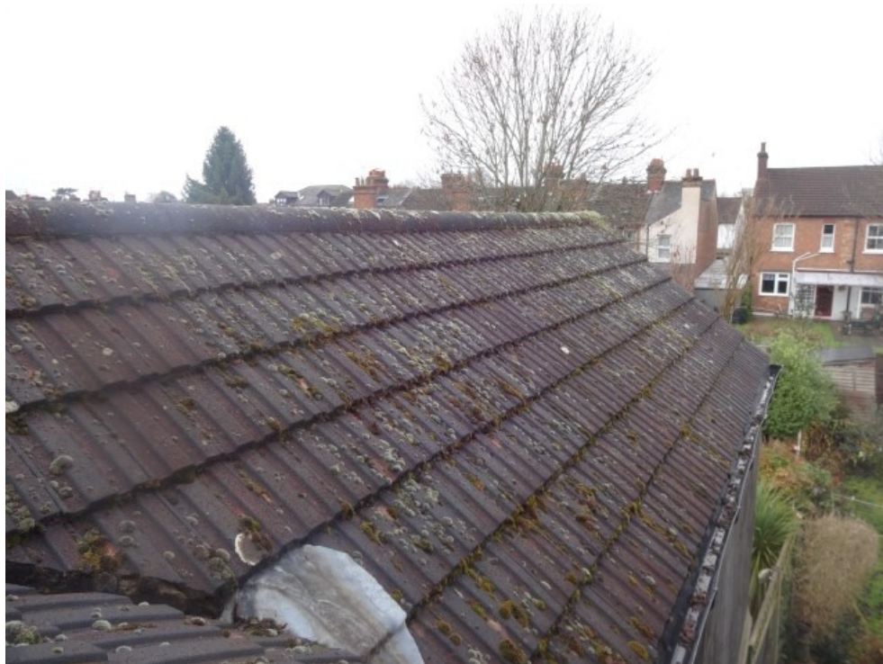
Rear roof over Bedroom 4
