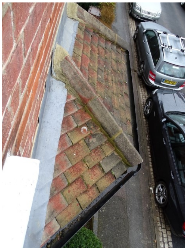
Roof to sitting room porch roof
