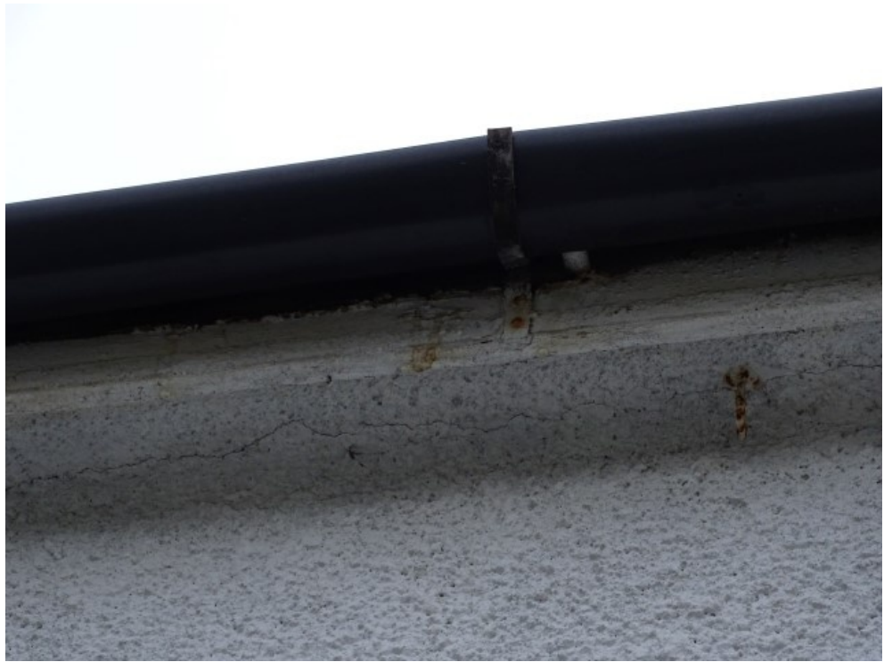
Rear gutter to main house
