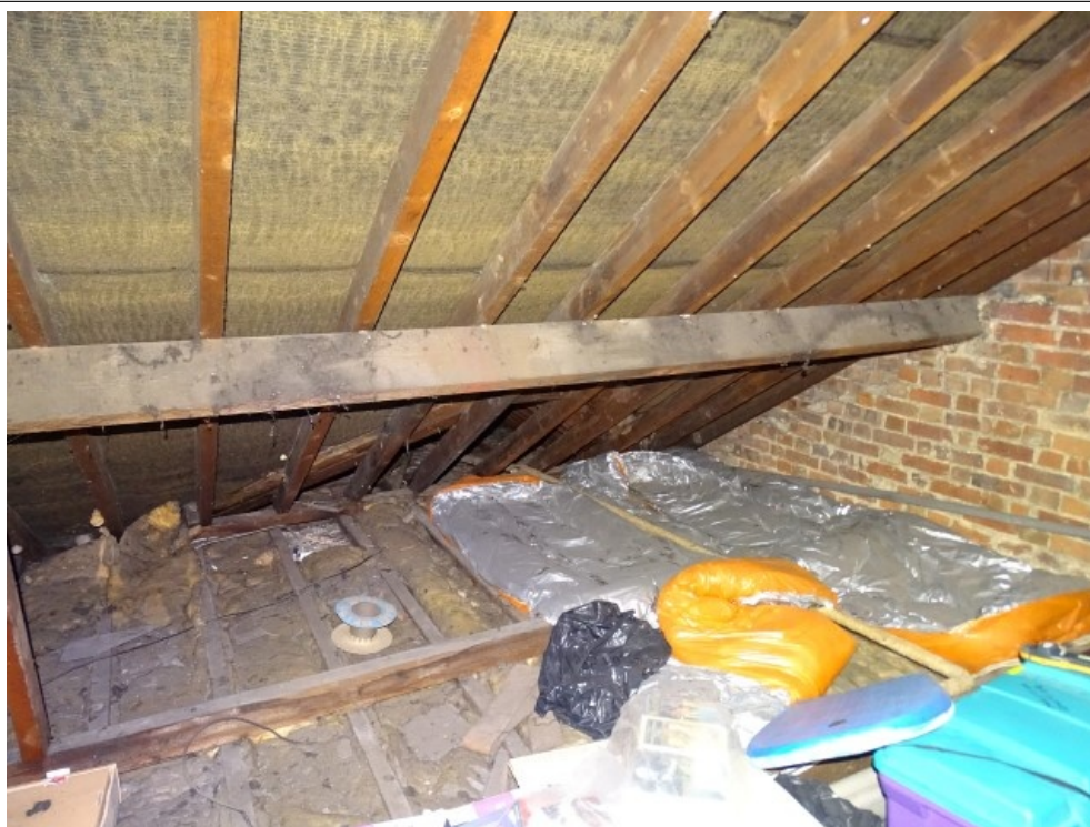
General view of roof structure
